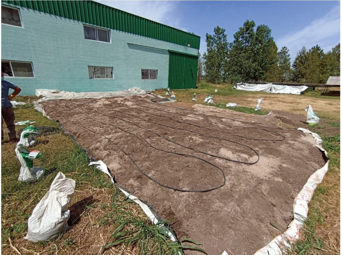
Figure 3. Drip tape installation in the solarization substrate
